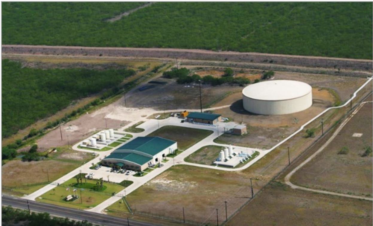
To increase water supply, BPUB is pursuing the expansion of the Southmost Regional Water Authority's facilities treatment abilities.
