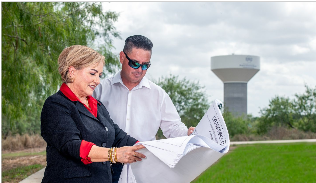
Marie Leal, Director of Water/Wastewater Engineering & Capital Planning, and David Vera, Field Technician, stand before the new Elevated Storage Tank.
