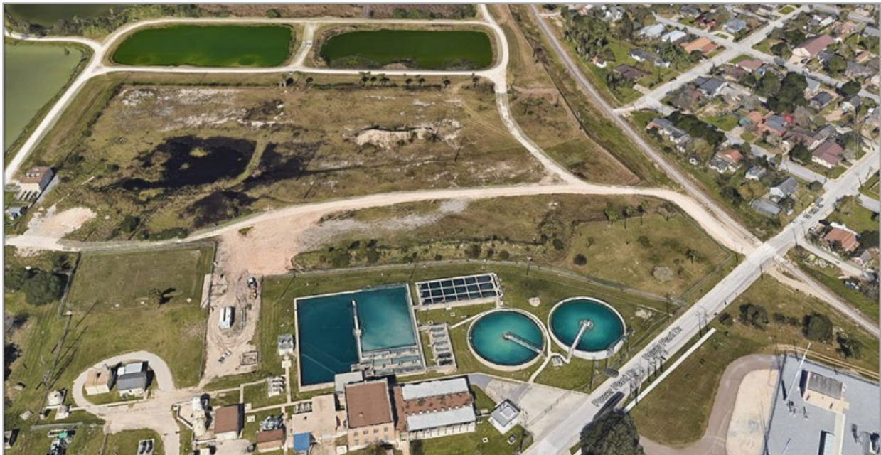
An aerial view of Water Plant 1 and the Silas Ray Power Plant.
